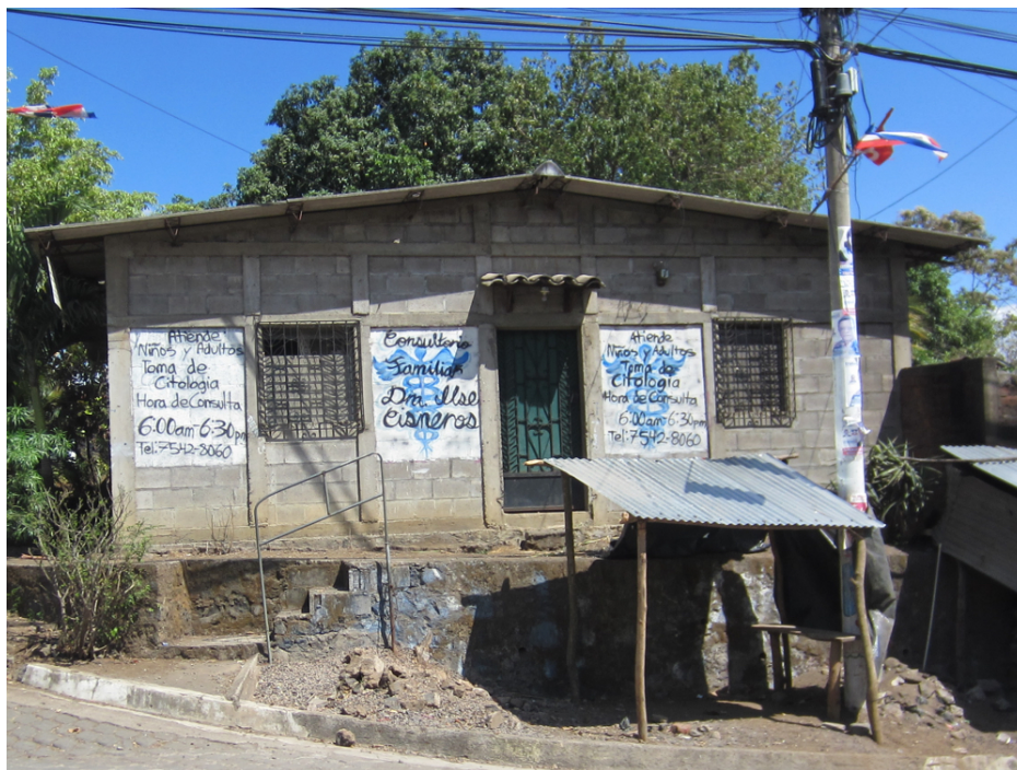
Figure 4.1. Façade of private clinic in small town announcing hours and services.
